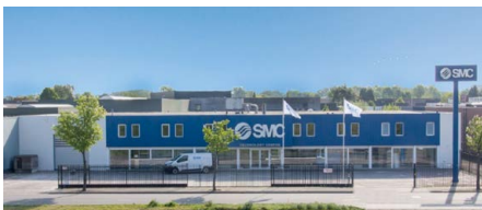
Technology Center Eindhoven
